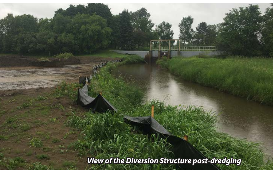
Sedimentation dredging of the Diversion Channel
