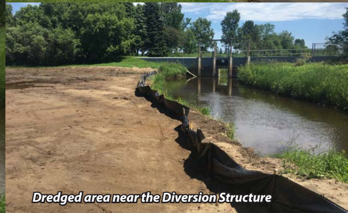
Sedimentation dredging of the Diversion Channel
