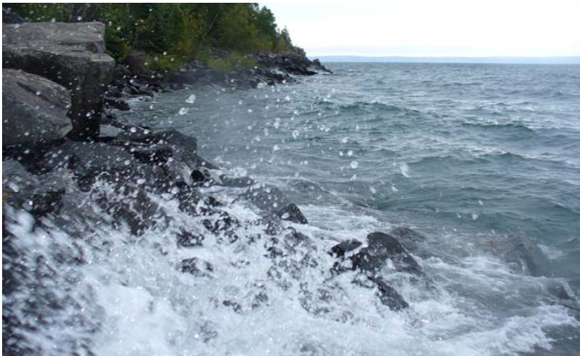
Rip Rap at Silver Harbour Conservation Area
