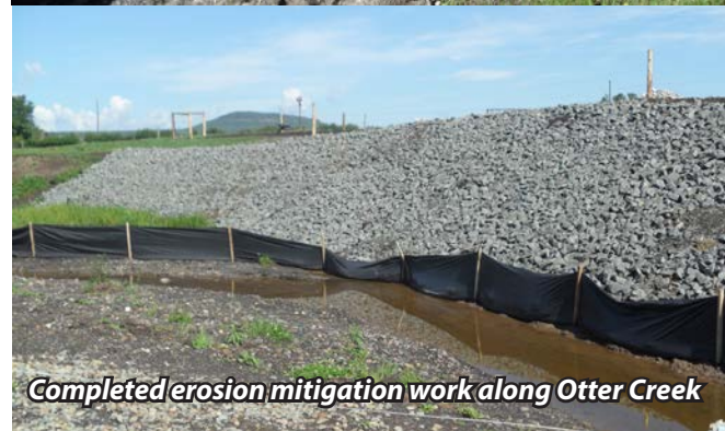
Cattle crossing work being completed along Oliver Creek
