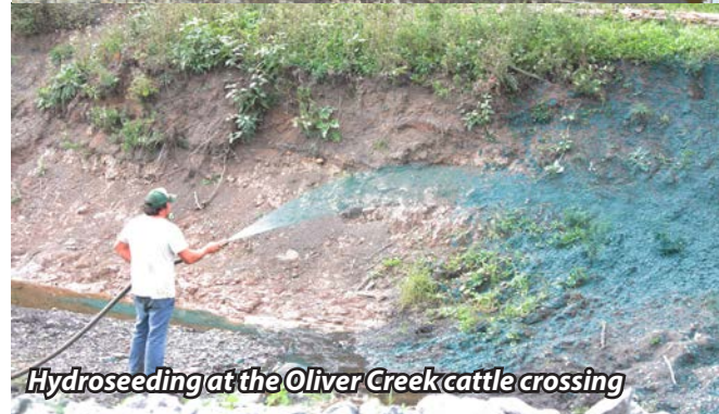
Completed erosion mitigation work along Otter Creek
