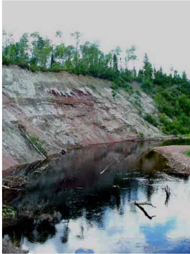
Figure 13: Bank Failure Further Upstream (LRCA 2009)
