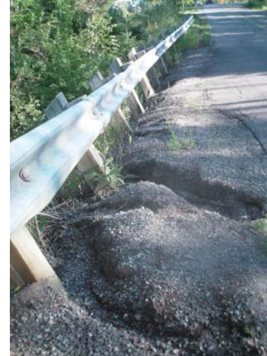
Downstream (west side of road)
