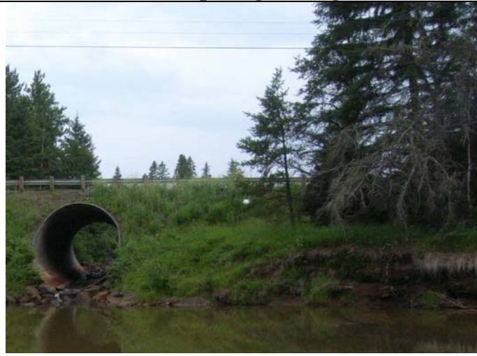
C: 2010 Culvert Opening to Large Pool Photo
