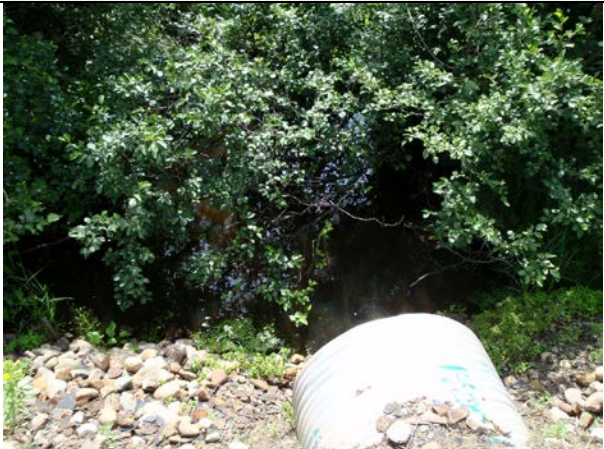
E: 2010 Culvert Downstream Photo
