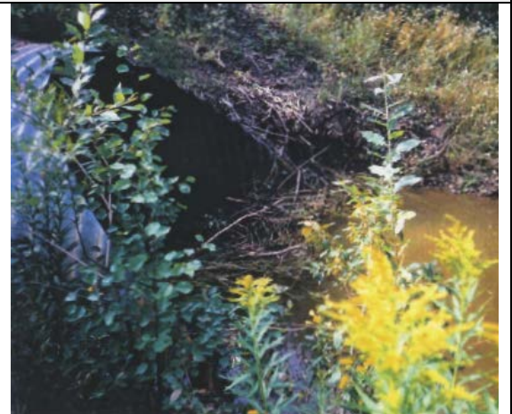
F: 1996 Culvert Photo, Facing Downstream
