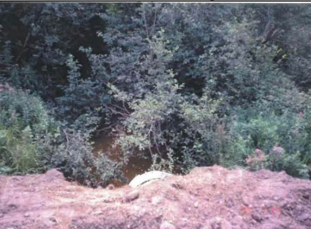
F: 1996 Culvert Photo, Facing Downstream
