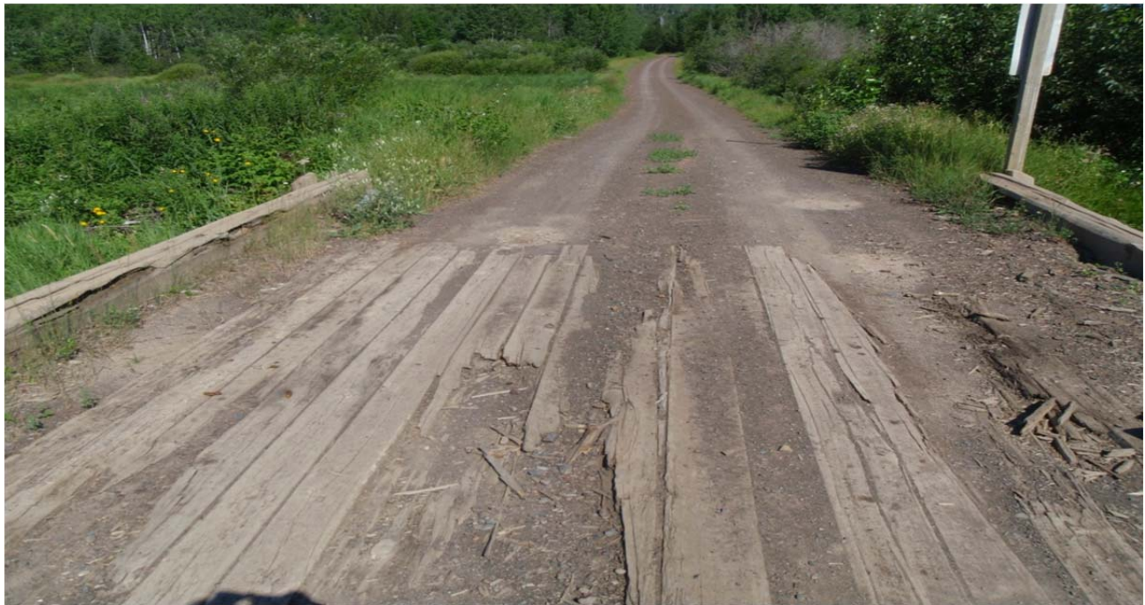
Figure 12: Degrading and Splintering Wood on Deck of Bridge 6
