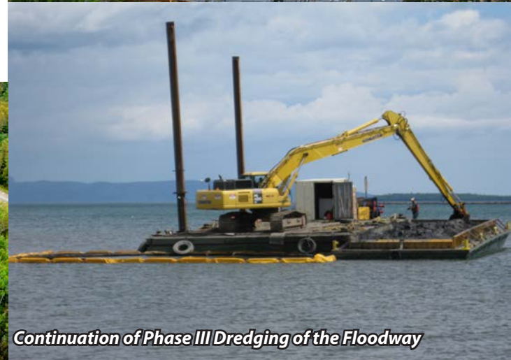
Phase III Dredging of the Floodway
