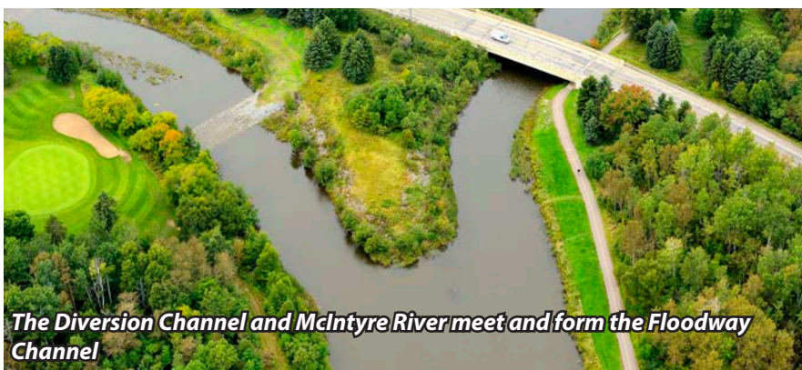
Continuation of Phase III Dredging of the Floodway
