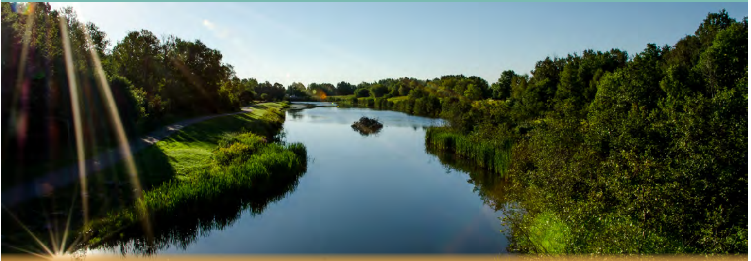
Neebing - McIntyre Floodway - widened, deepened Floodway Channel
