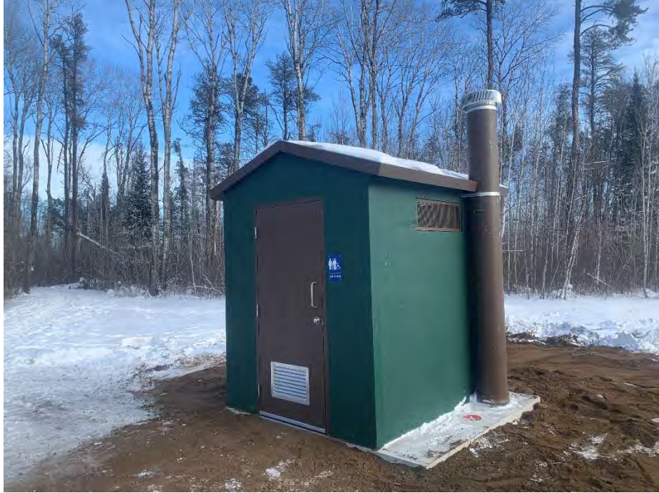
Photo 7: Installed AODA Outhouse at Cascades Conservation Area.
