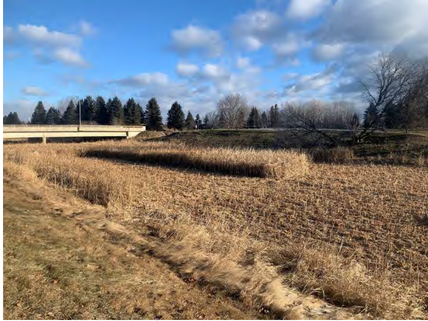
Photo 2: Ford St Section from Diversion Structure to Redwood Ave Bridge, during cutting process.
