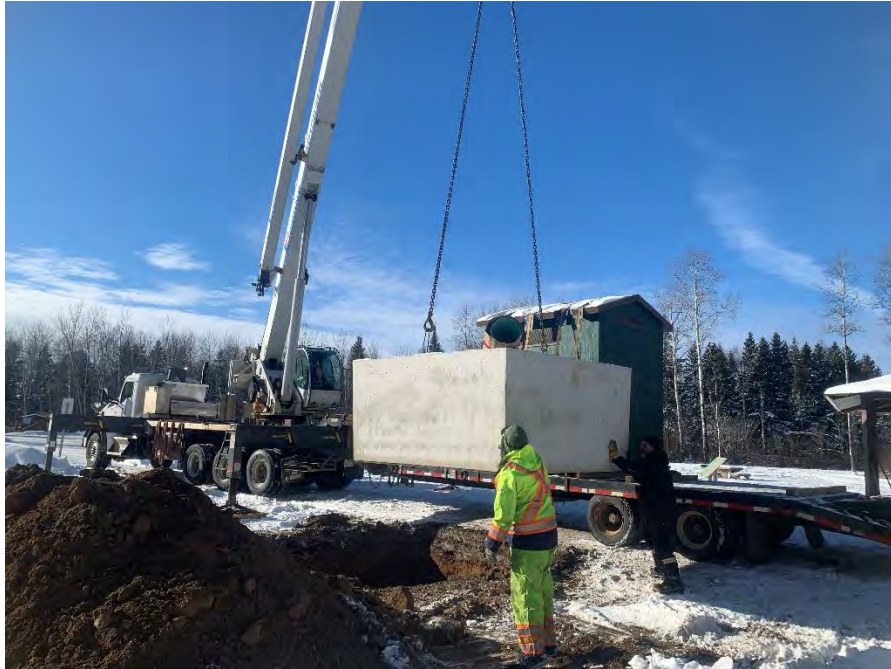
Photo 5: Crane Lowering holding tank into place.
