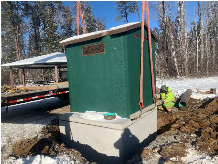
Photo 6: Top portion of unit being installed onto holding tank.
