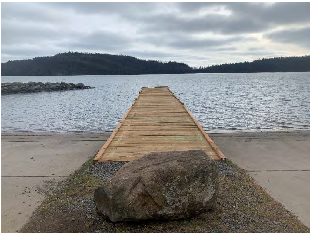
Photo 8: Little Trout Bay Dock Re-Decking and Rock Placement
