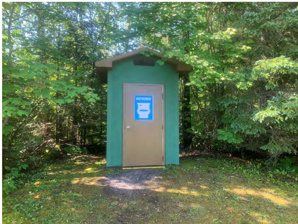
Photo 6: Outhouse Refurbishment Example
