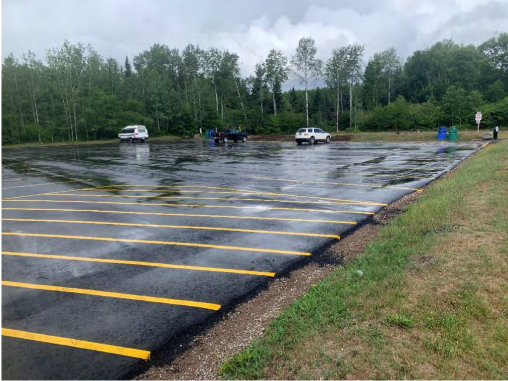
Photo 3: Cascades Parking Lot Paving
