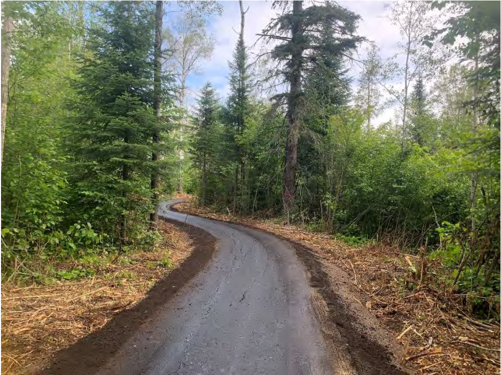
Photo 2: Cascades AODA Trail Paving
