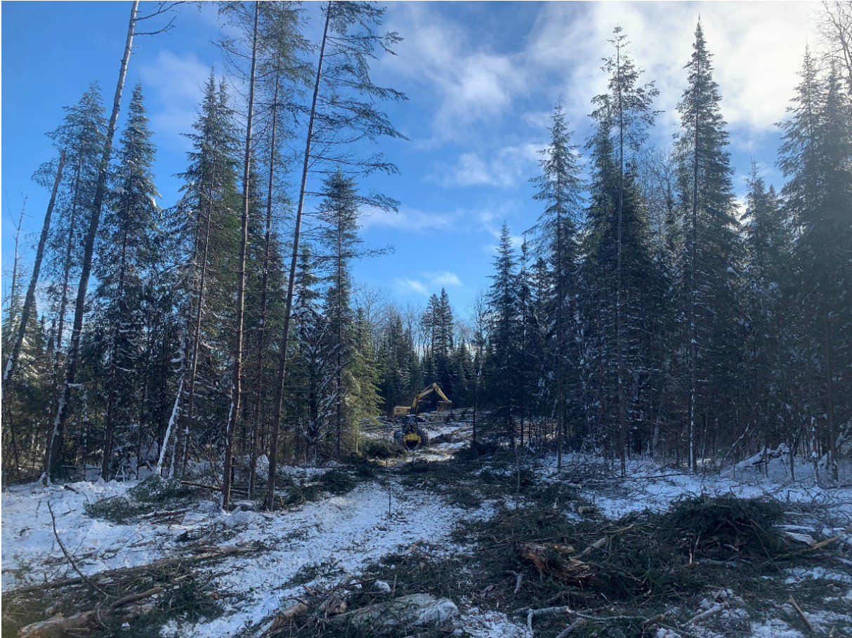
Photo 2. From cut line towards staging area, ground view.
