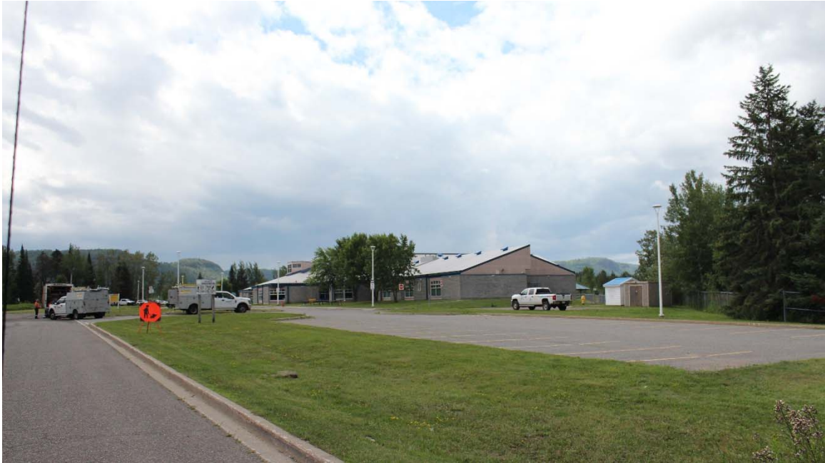
Figure 5: Nor'Wester View Public School
