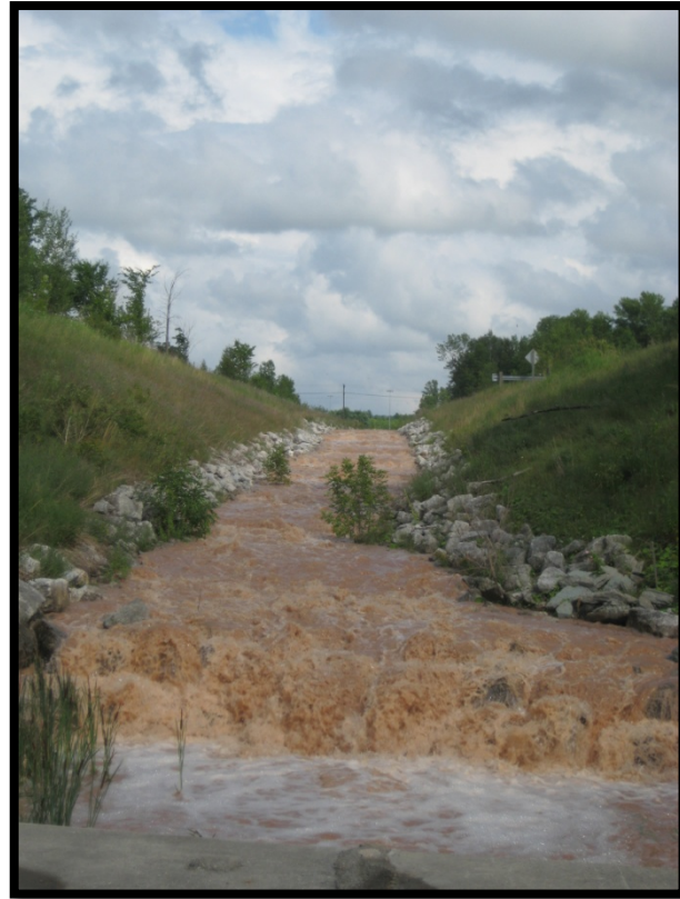
Figure 4: Under high flows, municipal drains and storm sewers can rapidly move contaminants toward a surface water intake. (SGSNBP Source Protection Region)
