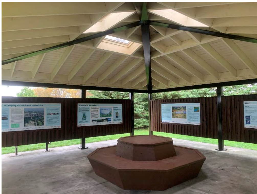
Photo 5: Mission Island Marsh Pavilion Refurbishment Interior
