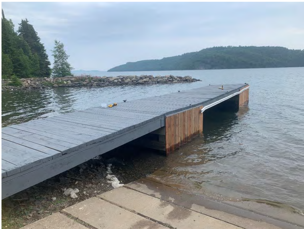
Photo 1: Little Trout Bay Dock Refurbishment
