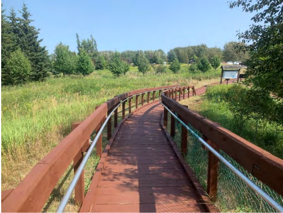
Photo 7: Mission Island Marsh Boardwalk Refurbishment
