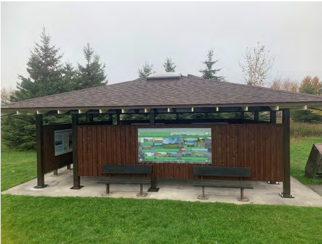
Photo 4: Mission Island Marsh Pavilion Refurbishment Exterior
