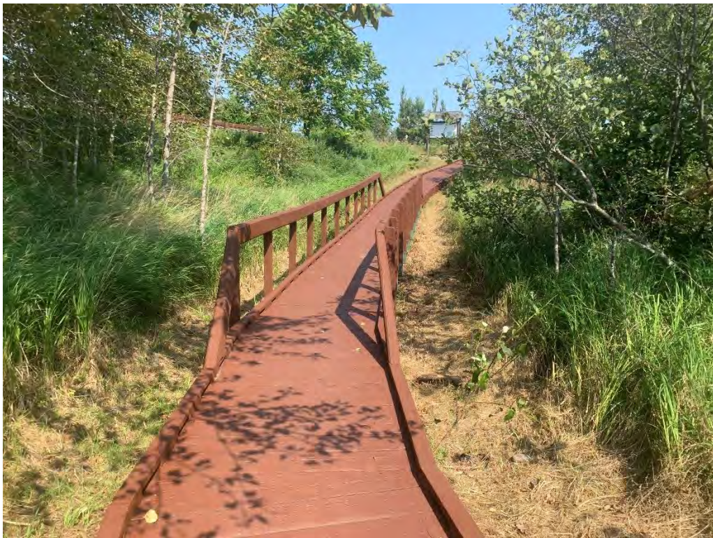
Photo 8: Mission Island Marsh Boardwalk Refurbishment
