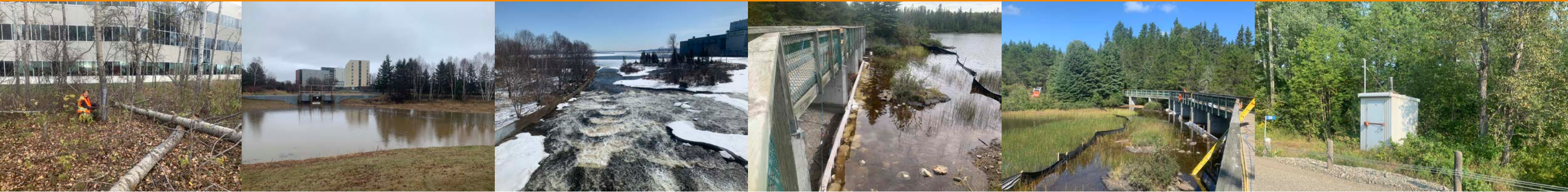
Photos (left to right): protecting trees from beavers along the Floodway; the Diversion Structure during spring freshet; the mouth of the Current River during high flows; major repair work on the Hazelwood Lake dam; Corbett Creek Streamflow/Precipitation Gauge Station.
