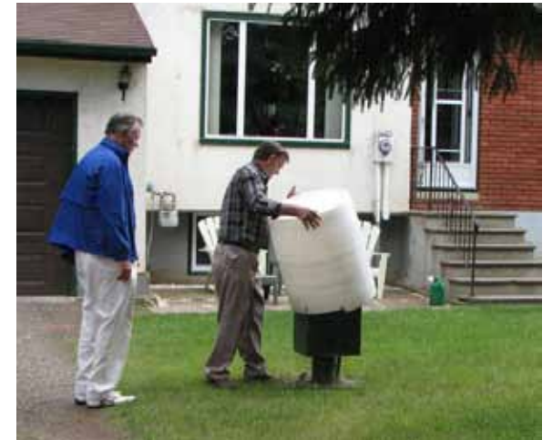
Committee Members, pictured above, examine a Municipal wellhead in Rosslyn Village.
